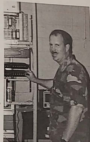
TSgt. Douglas Carrell works on installing a new Giant Voice System at Cannon AFB, N.M.
